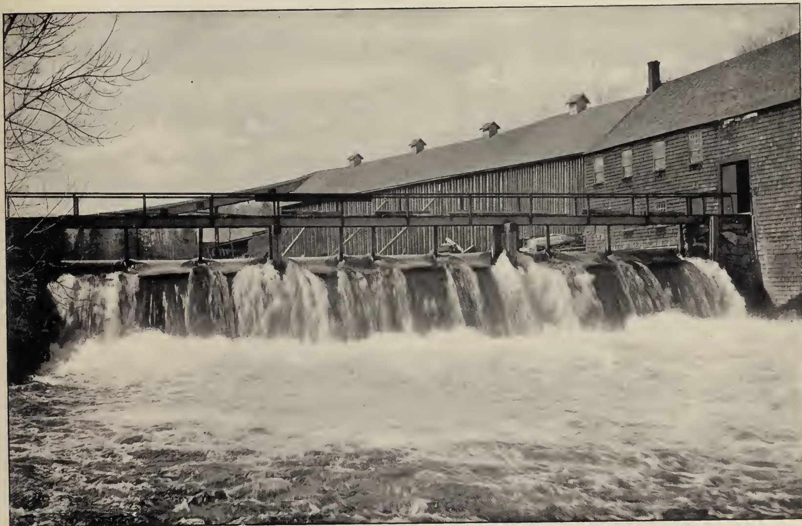
DAM NO. 4, OWNED BY THE HOLLINGSWORTH & WHITNEY CO.—FALL 15.90 FEET. See Page 35.
